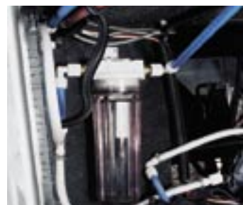
The water filtration system provides safe clean drinking water through all the water lines.
