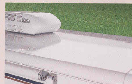
One-year-old Winnebago Industries fiberglass roof
