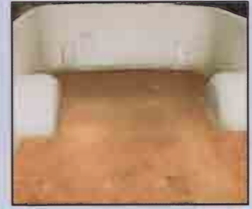
Wood flooring installed and sealed with fiberglass prior to carpeting.
