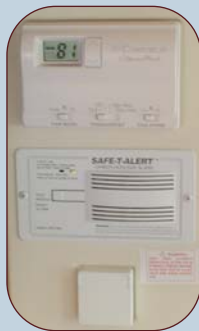
Furnace & A/C Control
